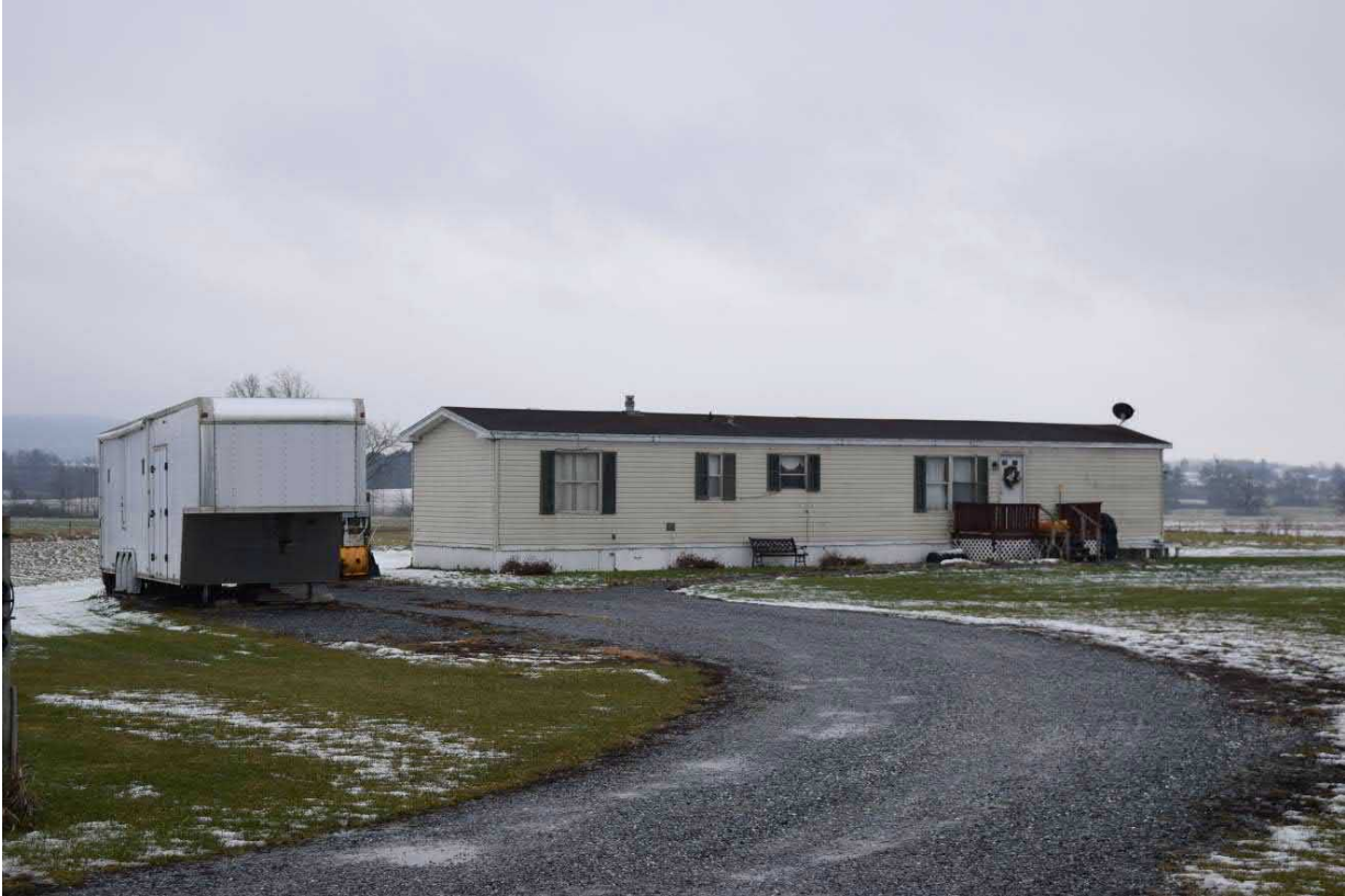
Photo 15. View of Structure 3, facing southeast.
