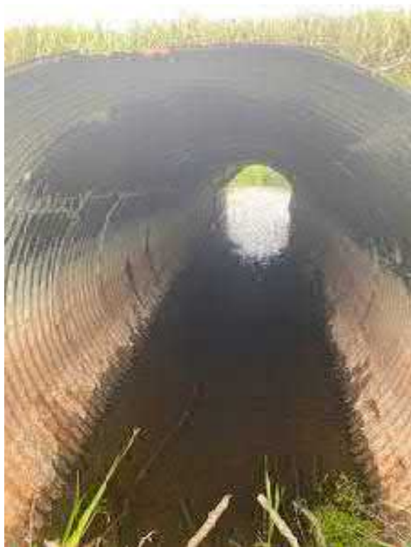
Photo 6: Culvert Interior Dated: 06/29/2021
