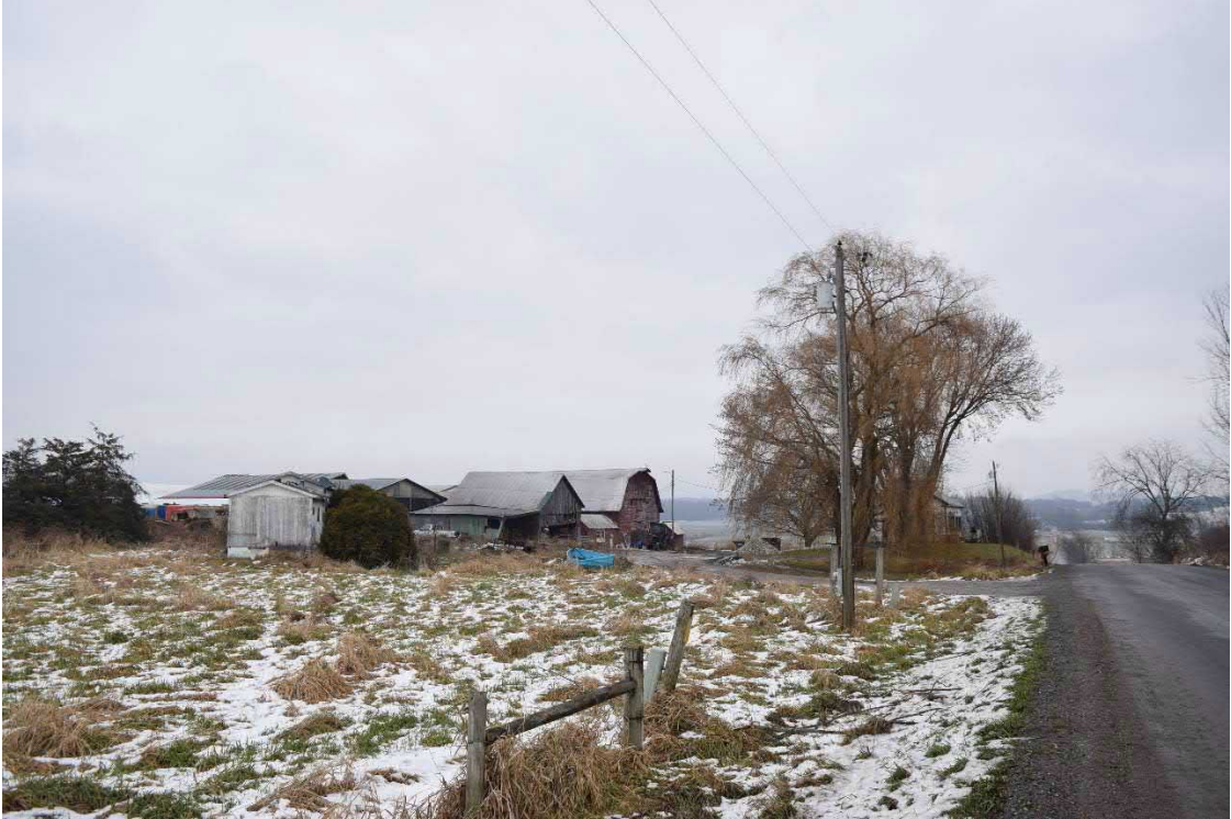
Photo 10. View of barn-complex associated with Structure 2, facing northeast.
