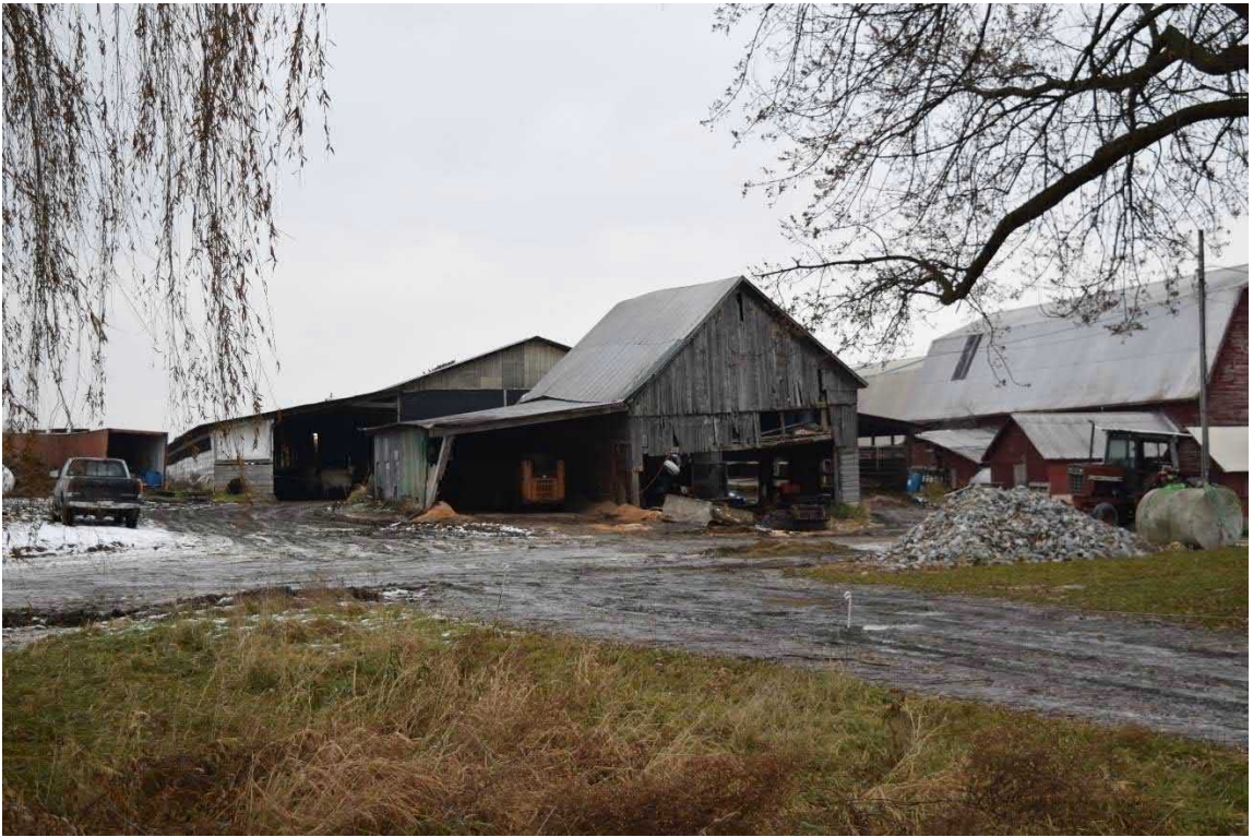
Photo 13. View of barn associated with Structure 2, facing north-northeast.
