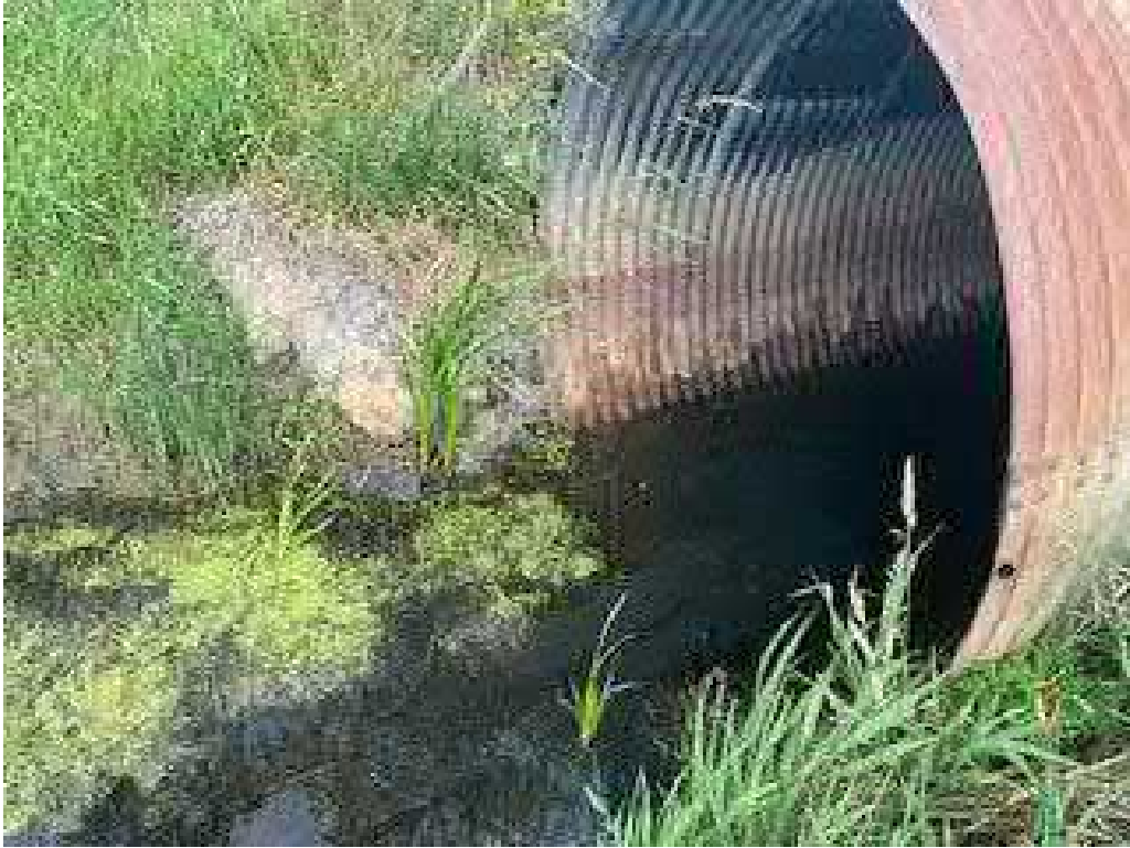
Photo 7: Culvert Downstream Invert Out Dated: 06/29/2021
