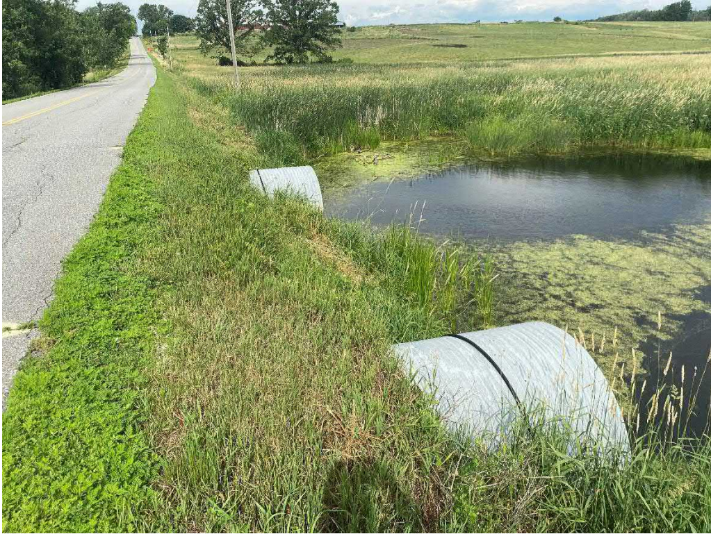
Photo 1: Roadway Looking Westbound Dated: 07/14/2021
