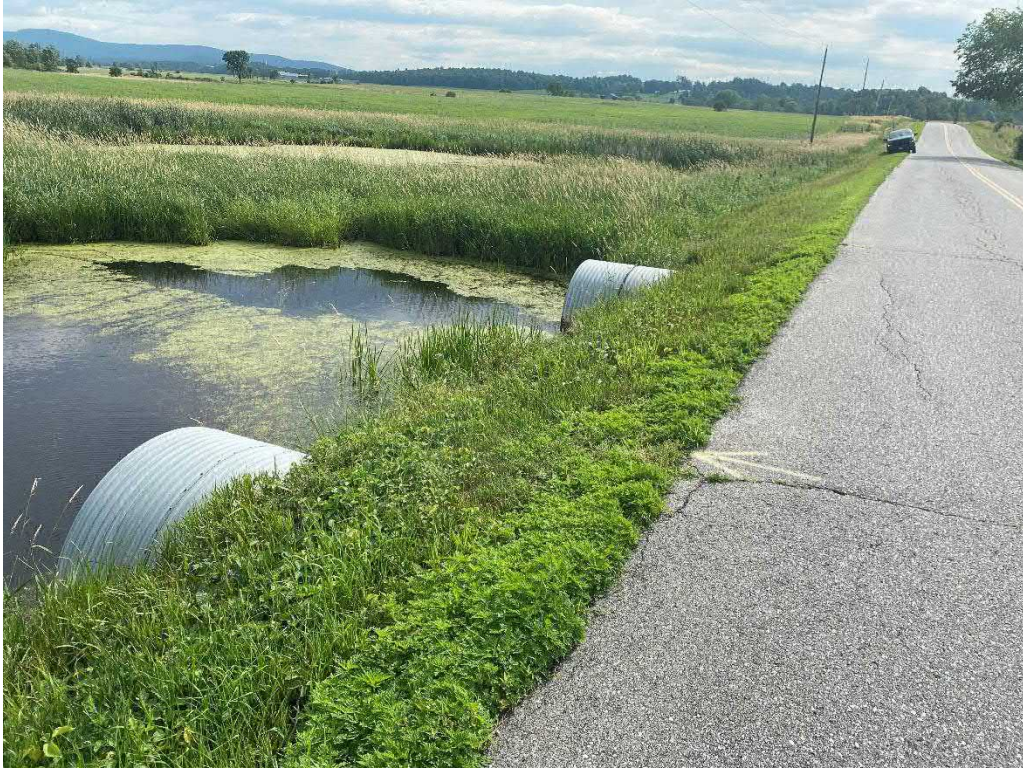
Photo 3: Culvert Upstream Inlets Dated: 07/14/2021
