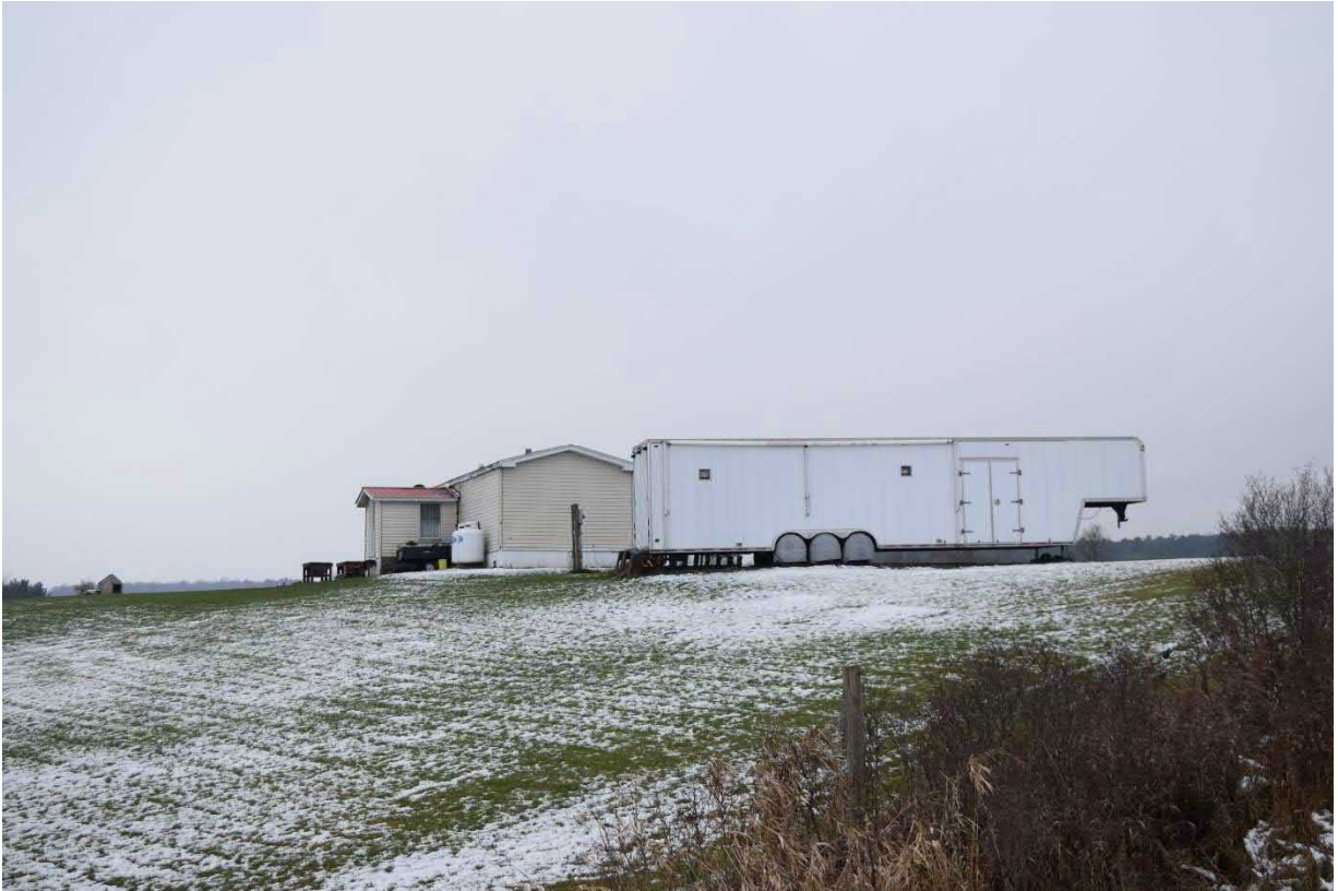
Photo 16. View of Structure 3, facing southwest.
