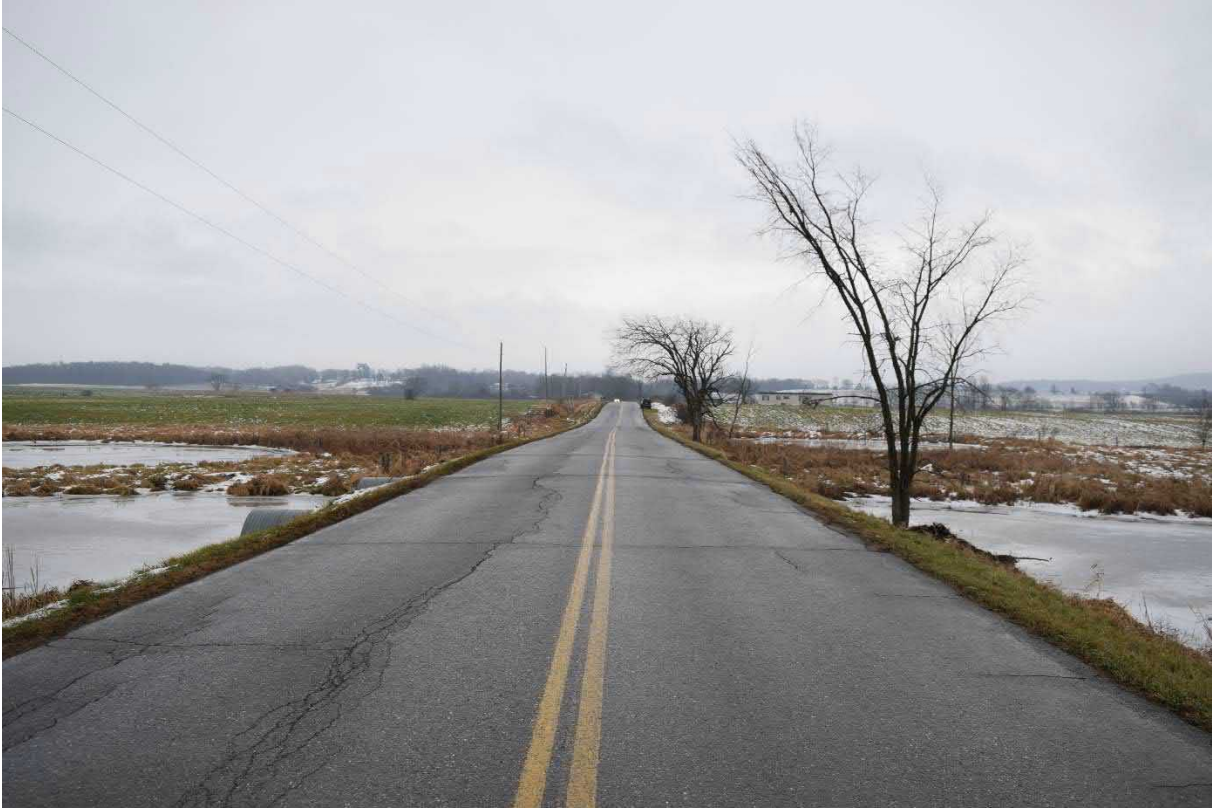
Photo 5. View of Structure 1, looking east-northeast.
