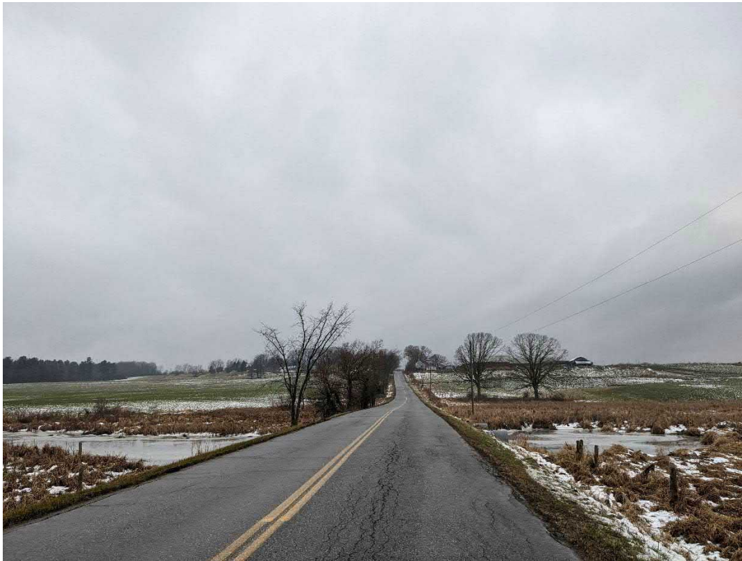
Photo 1. View of Middle Road, facing west-southwest. Structure 1 seen in foreground and Structure 2 seen in background at right.
