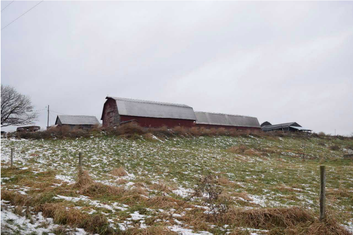
Photo 11. View of barn-complex associated with Structure 2, facing northwest.
