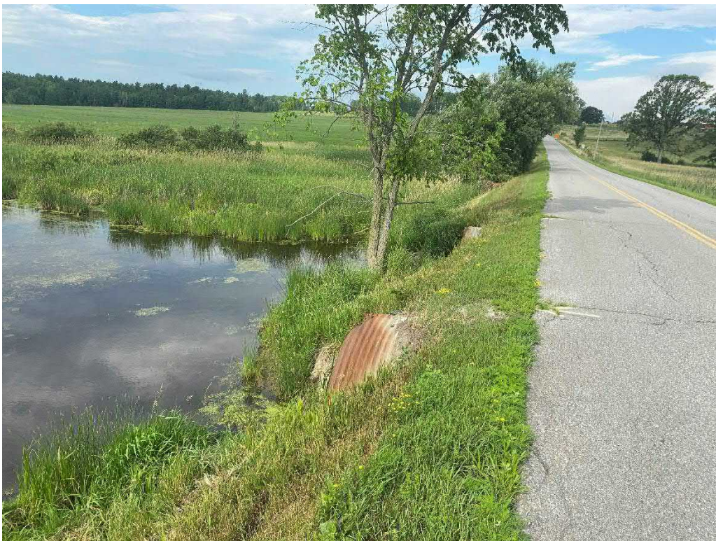
Photo 4: Culvert Downstream Outlets Dated: 07/14/2021
